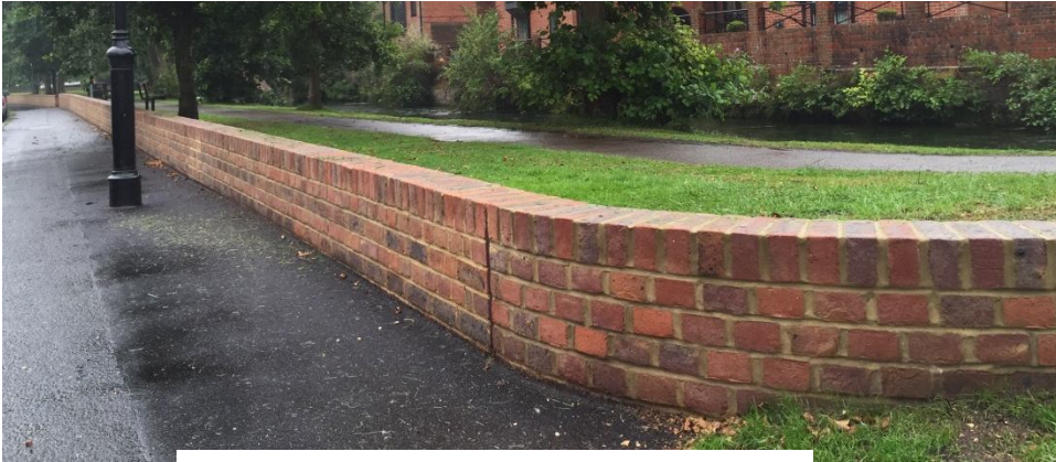
Water Lane Flood Defence Wall
