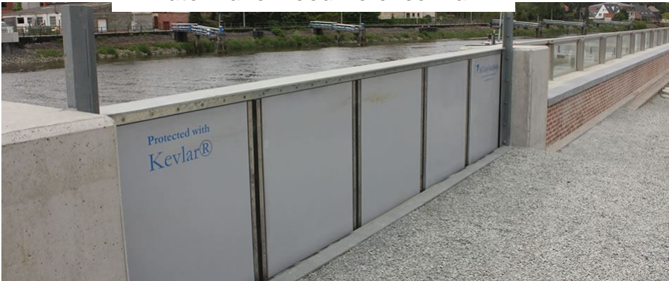
Typical Flood Gate
