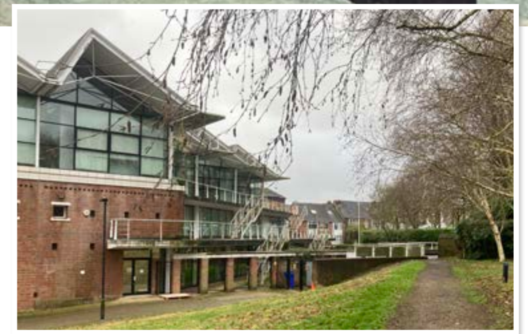
Existing photograph of centre of Carfax site
