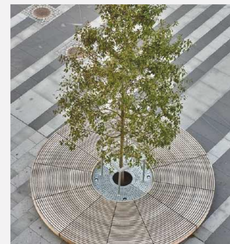
Improved paving and tree protection
